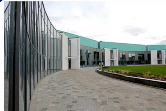
Temporary modular school building
